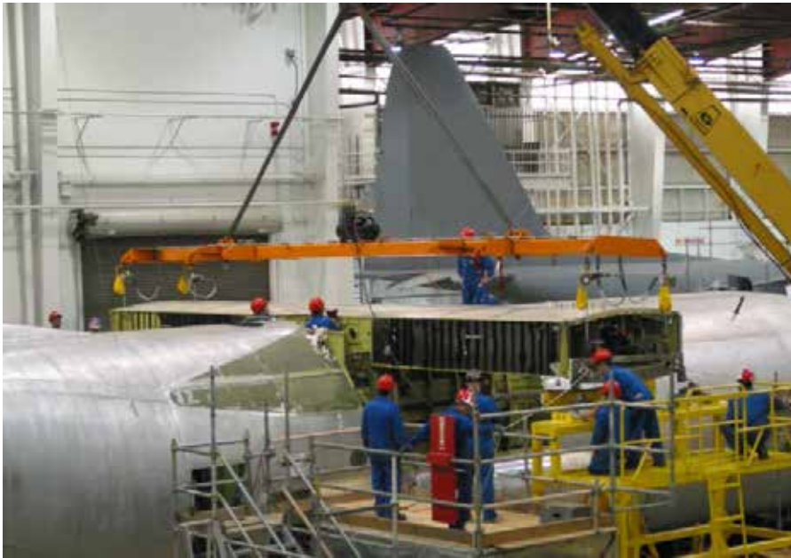
Figure A-3 Positioning a C-130 Centre Wing
